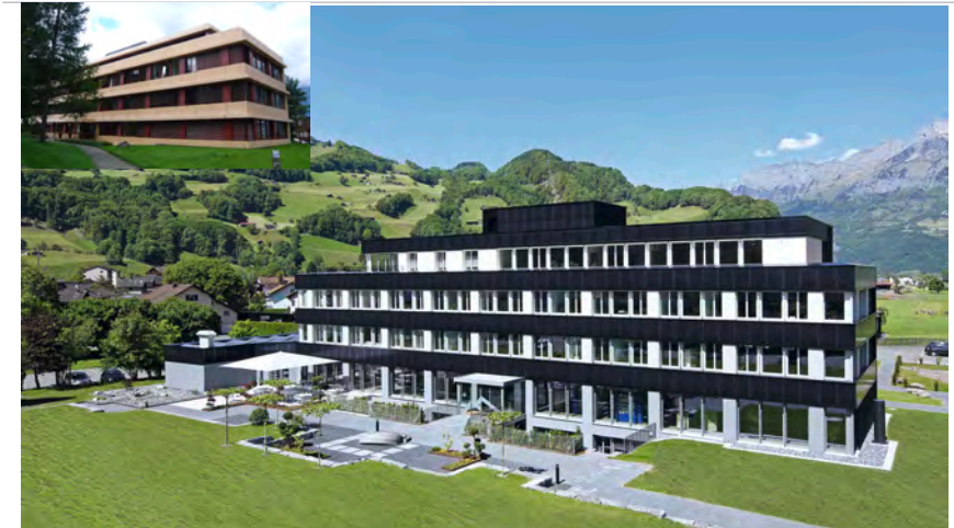
Flums: Plus energy renovation of an office building – built 1984 / renovation 2014 Photovoltaic integrated on the facade (414 m 2 ) and flat roof (403 m 2 )
