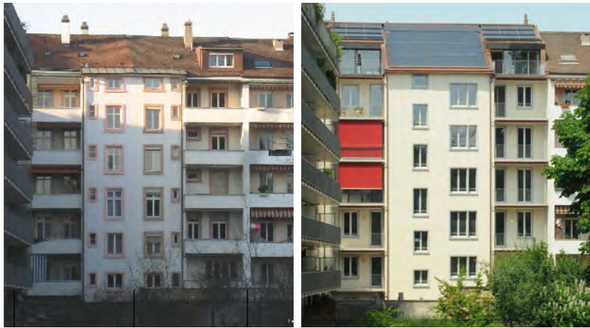
Bale, Feldbergstrasse: zero energy renovation – built 1896 / renovation 2009 Watt d'Or 2010 (BFE) category Reconstruction
