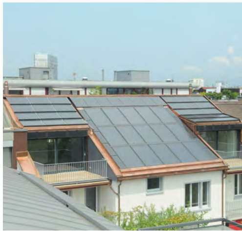
Bale, Feldbergstrasse: zero energy renovation Only 100 m 2 roof for thermic suncollectors and photovoltaic for 6 floor levels
